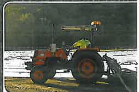
Fytofoam being applied - Tunks Park, North Sydney
